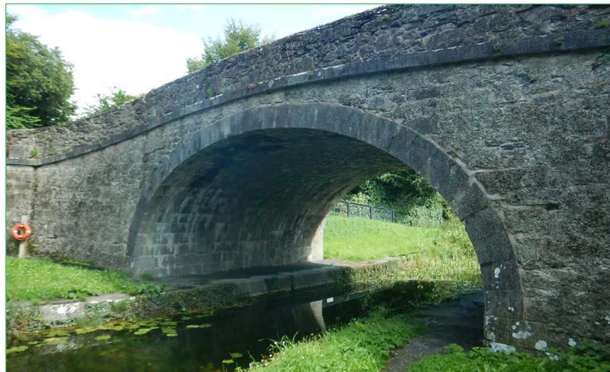
Figure 7-14 View of Connaught Bridge
