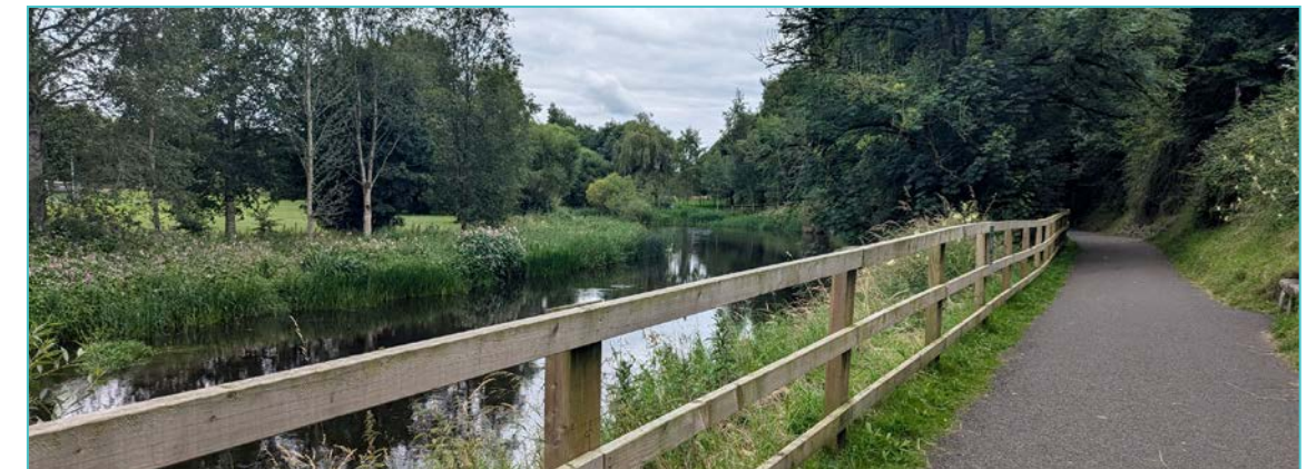
Figure 4-8 Footpath along River Liffey in Liffey Valley Park, Newbridge
