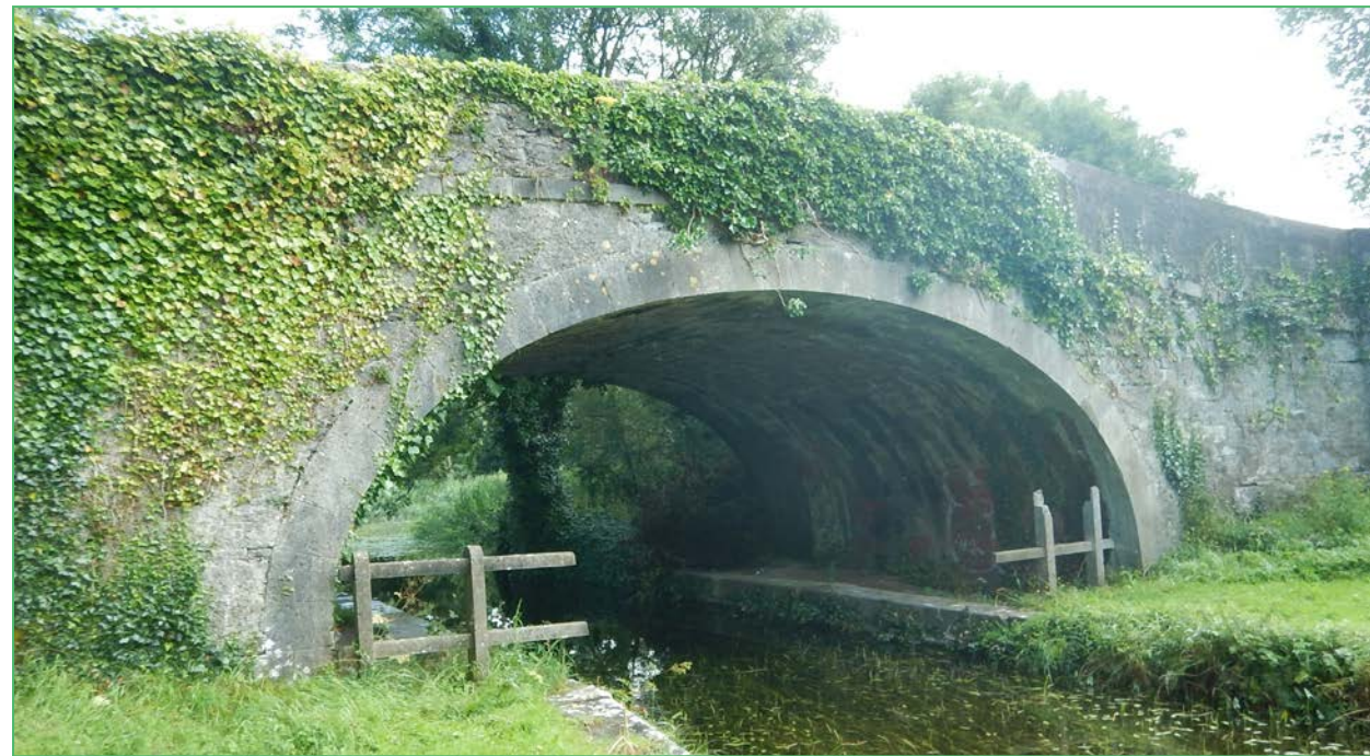
Figure 7-13 View of Limerick Bridge
