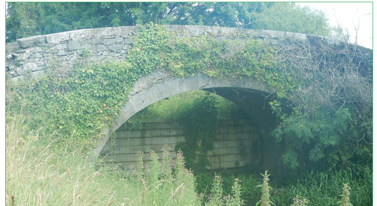
Figure 7-16 View of Tractor Culvert at Mooney Bridge (visible beneath Mooney Bridge)
