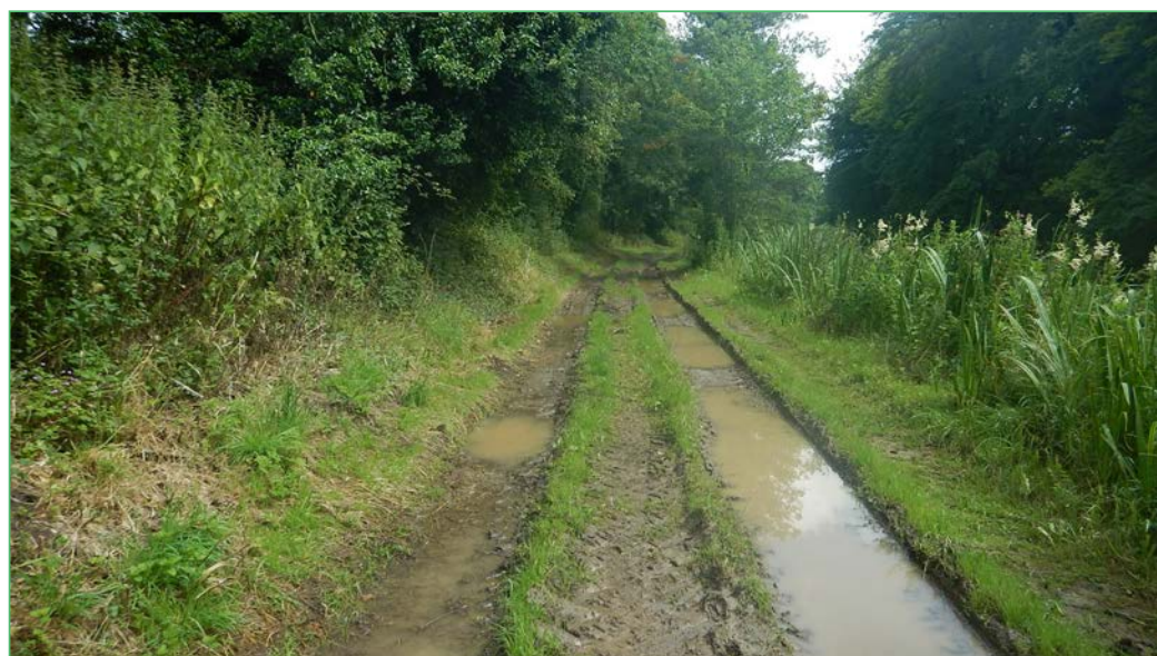
Figure 7-5 Photo showing wet path at central location of the Corbally Canal trail during site visit in July 2024
