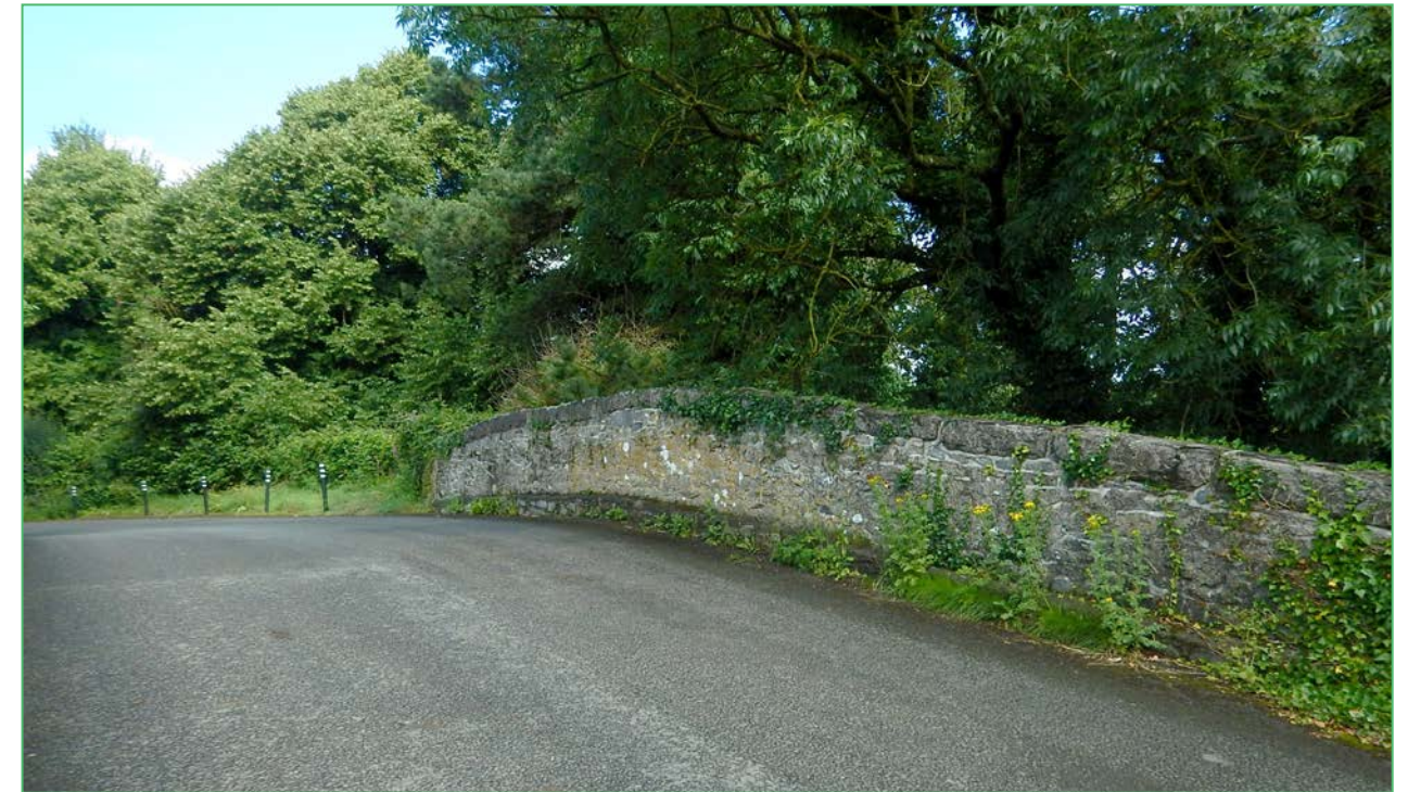
Figure 7-7 Existing bridge (Connaught Bridge) over Corbally Canal
