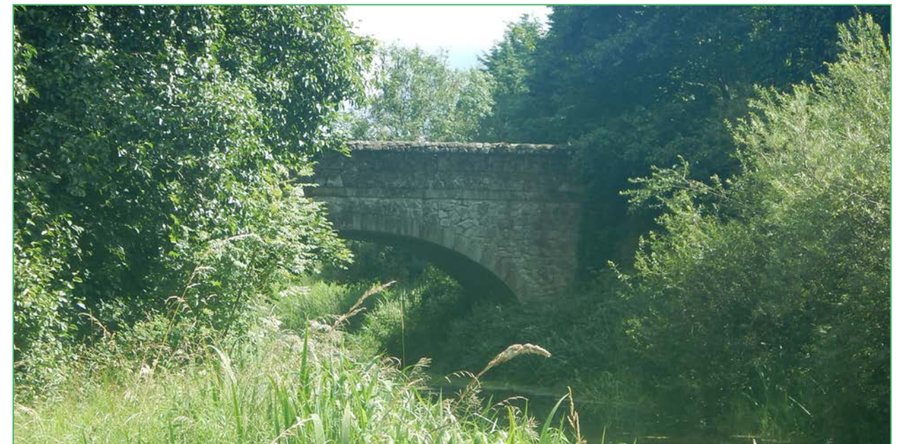
Figure 7-15 View of Hoare Bridge
